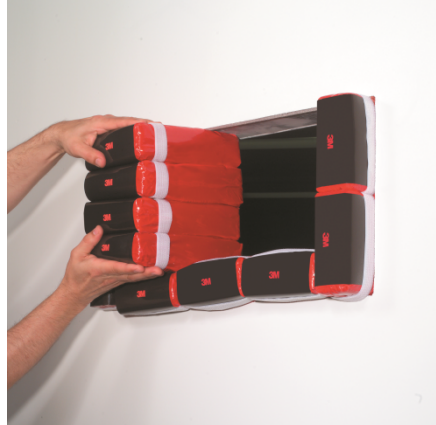
Figure 6.2.4. Installing fire barrier pillows. Photo courtesy of 3M
