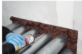
680 Figure 5.2.1. Fire rated foam application.
